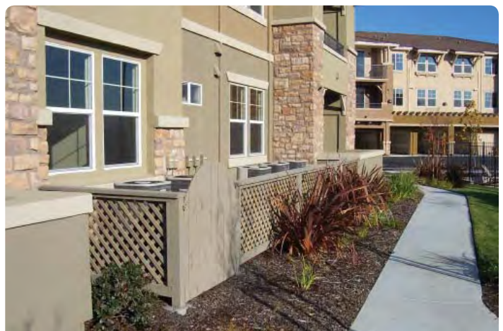
Air conditioner units screened behind landscaping and screen walls enhance the pedestrian environment.
