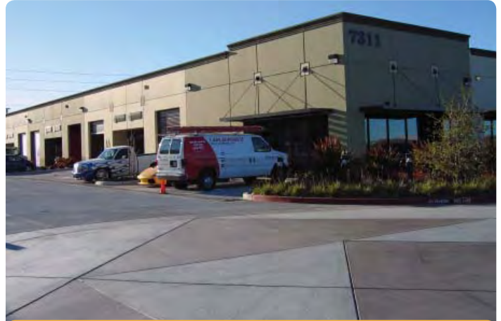
Service bays with roll up doors are oriented internally and away from the street frontage.
