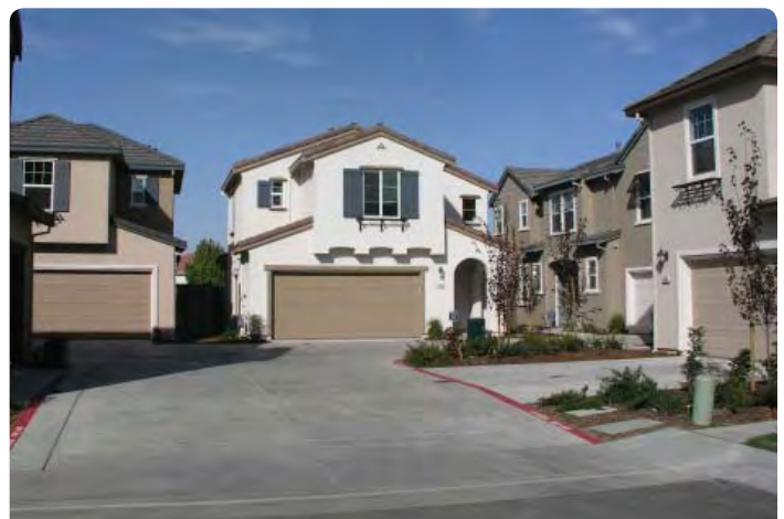
Score lines and a salt finish increase the visual interest of this motorcourt driveway.
